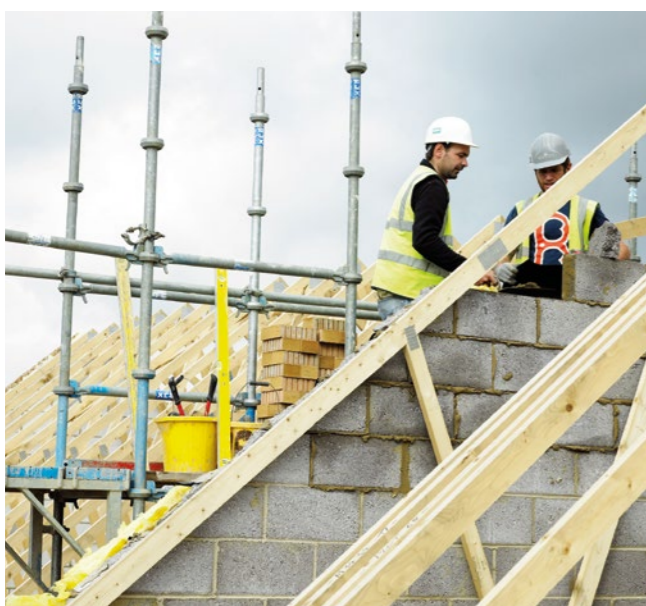
↖ New homes under construction.
