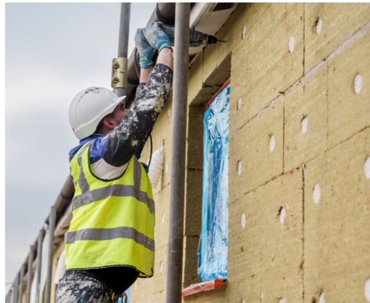
Retrofit investment at Barnstaple Court, Bristol
